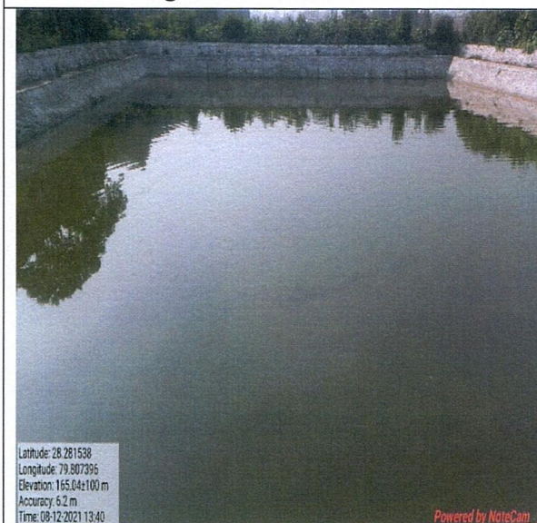
Figure 5 Treated effluent Lagoon
